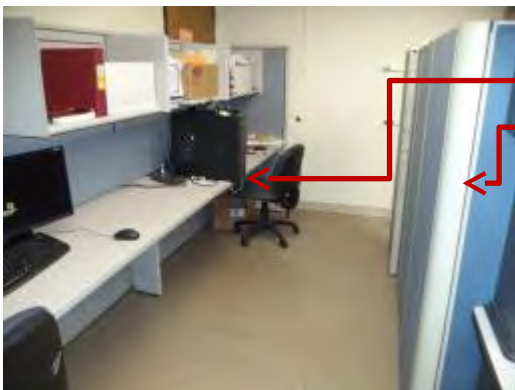
Grad offices located in aisle way to same lab, impeding egress
