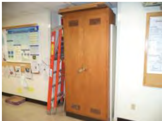
Storage placed in corridor due to lack of space
