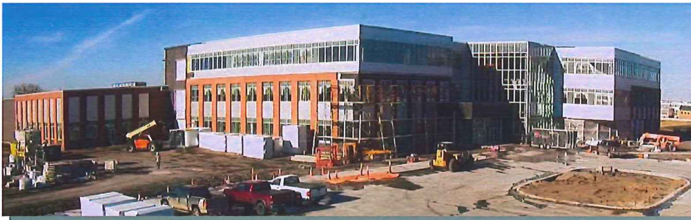
Peltier Complex Under Construction
